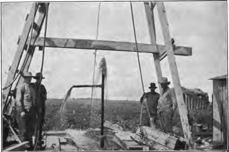
FIG. 145. Flowing Well, Just Struck, Trott Farm, Casselton Quadrangle. (Depth 418 feet. Flow at first, 4,000 barrels per day. Section 10, Township 140, Range 53.)
